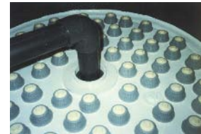
COLECTOR DE PLACA COLLECTOR PLATE WITH NOZZLES
