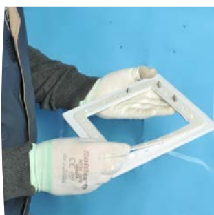
Place the seal over the flange
