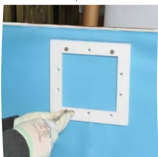
Screw the flange and hollow out the liner
