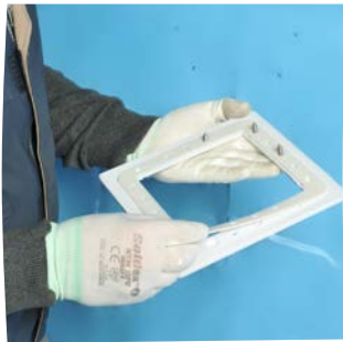
Place the seal over the flange
