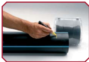
Machine the welding zone surface by means of a peeling tool, scraper or proper tool.
